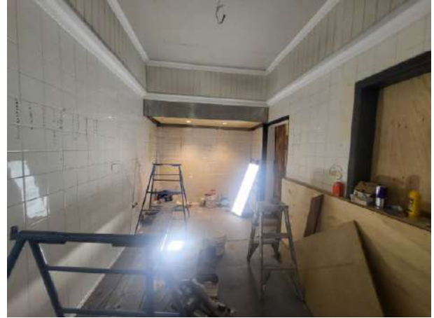
Area previously utilised as a Kitchen
