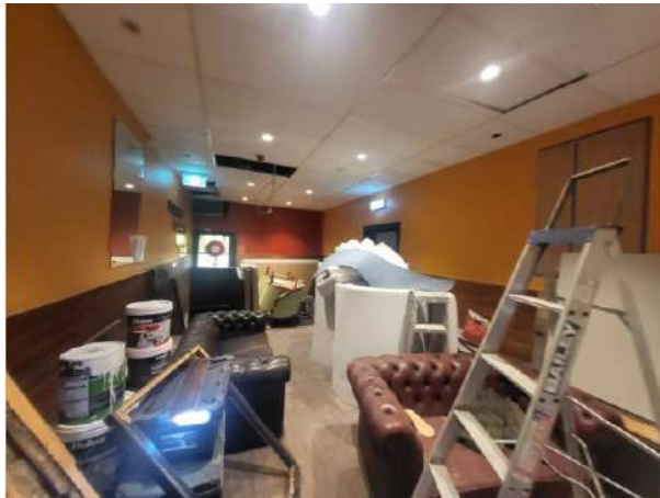
Large First Level Area
