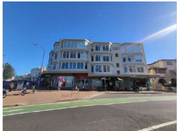
Subject Complex from Lamrock Place
